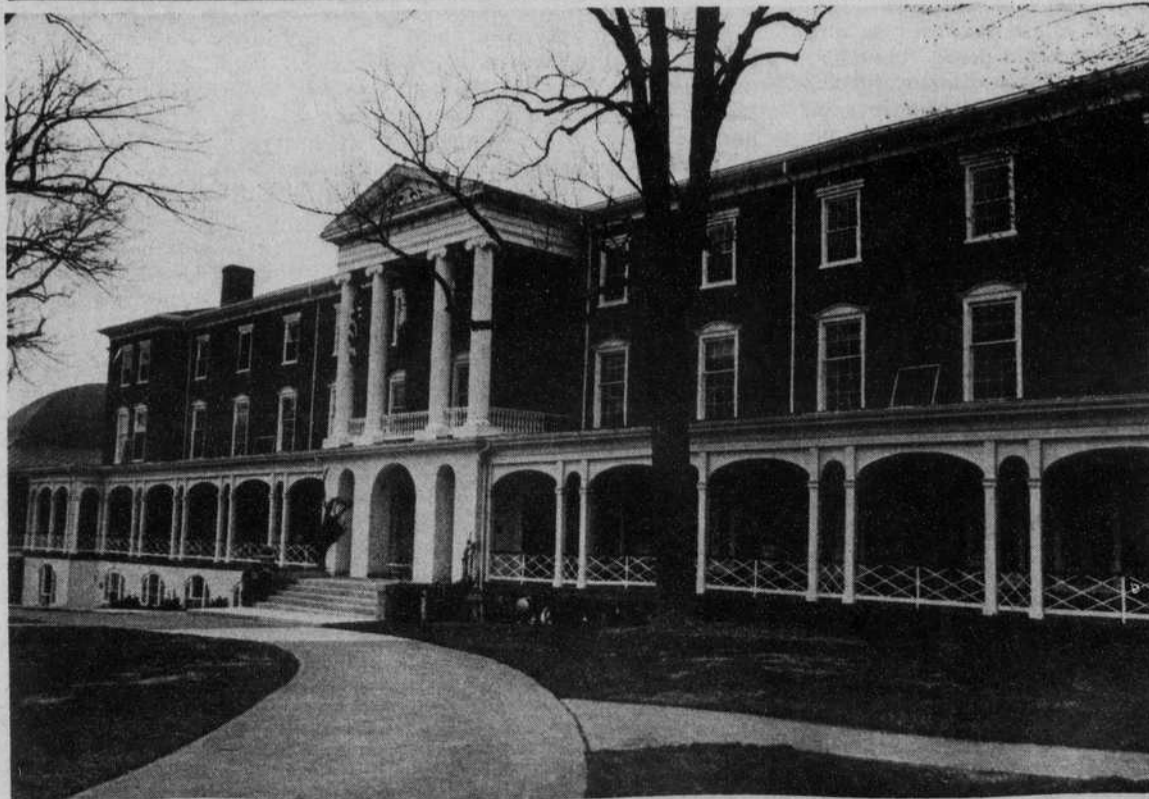
Main Building, closed for a year of renovations, will house 44 students in 1981-82.
