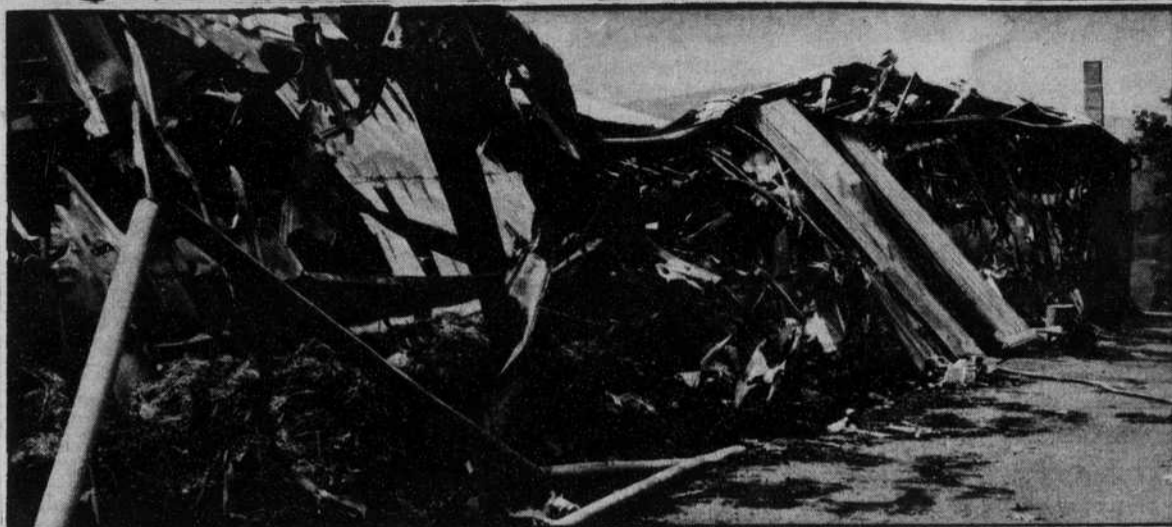
A July fire left the stables destroyed, although the indoor riding ring survived. Photo by Robin McCormick
