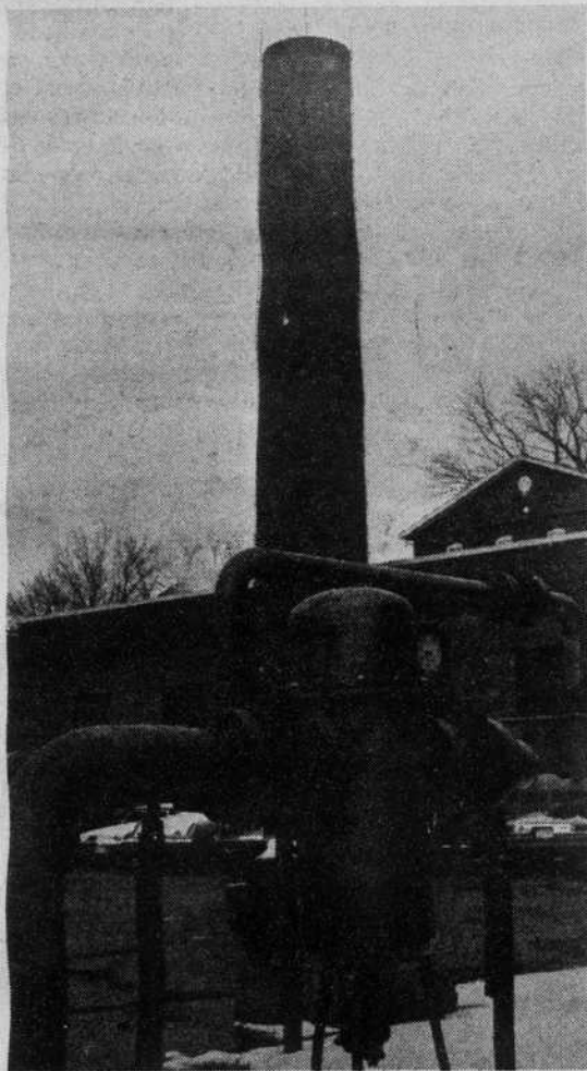
Hollins' "busiest and most expensive building," the power plant.
