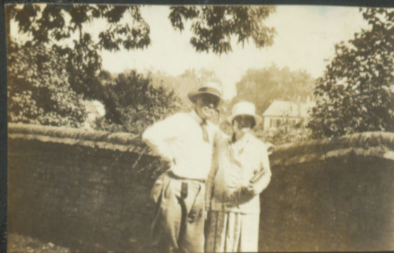
An old brick wall
